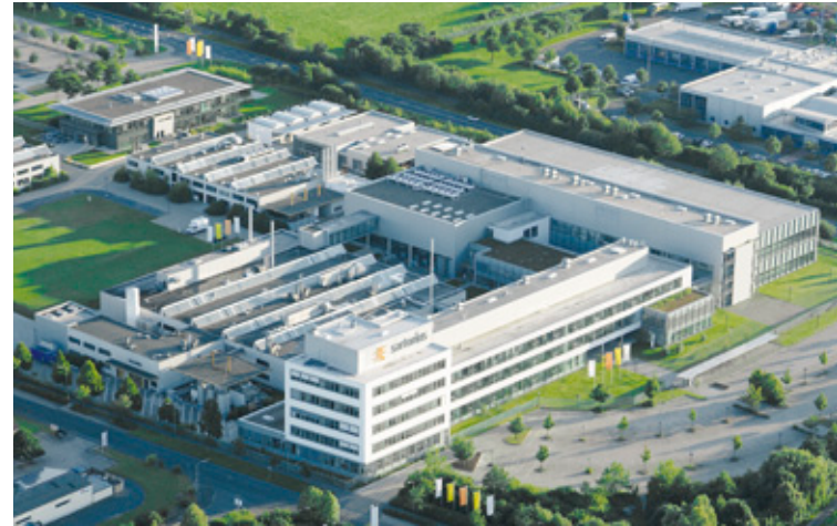
Sartorius Stedim Biotech plant in Goettingen, Germany
